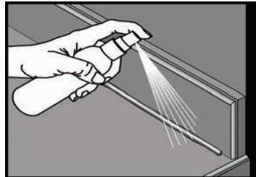
2.) Before tooling, spray MIST onto Silicone and the PERFECT BEAD TOOL to help smooth silicone bead during tooling. MIST also helps to keep excess silicone from adhering to areas where silicone is not wanted.
